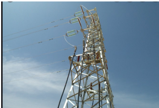
Image 9 – Inspection of cable termination and Insulators at tower
