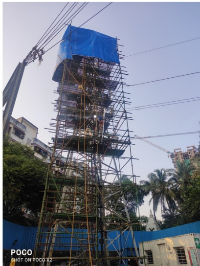
Image 8 - 110 KV Cable termination work at Tower
