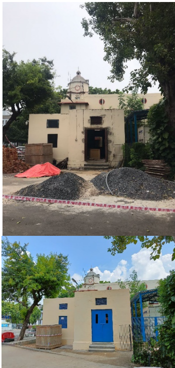
Fig. 12. Tata Power-DDL St Xavier substation in Delhi
