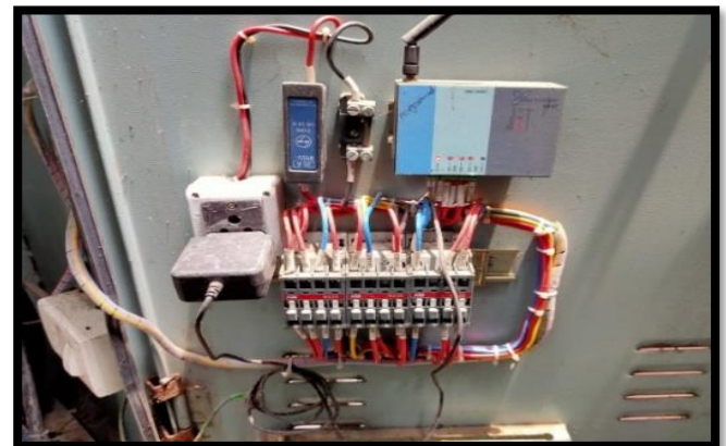
DTR LT HRC Fuse indicator at BBD Bag D/S O/T No.-2
